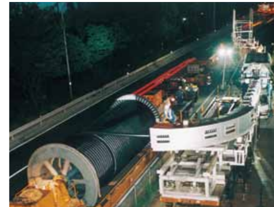
500kV XLPE cable installation work in Shinkeiyo Toyosu Line in 1996
