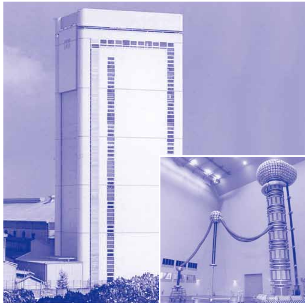
VCV tower in Osaka Works
