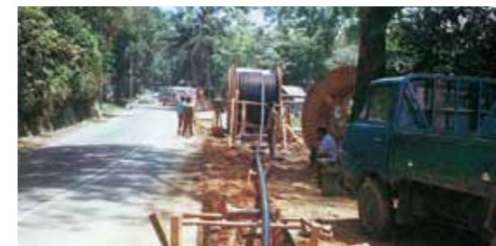
Direct burial cable installation work in Singapore
